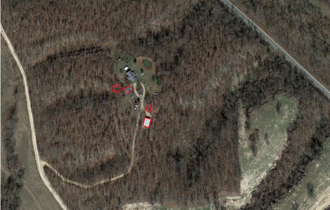
Image of the new buildings after the work has been completed (Image Date March 2017)
