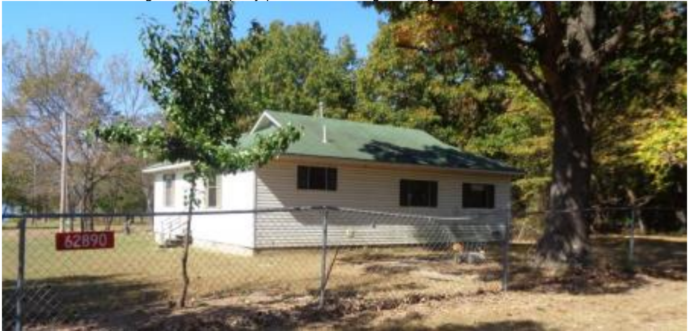
Image of the property prior to the changes (Image Date - 10/29/2015)
