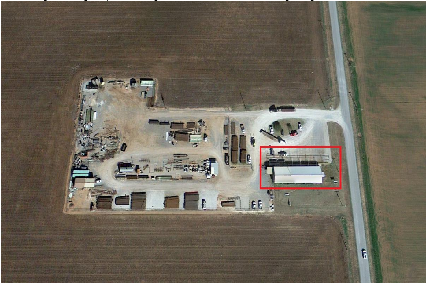
Image showing the parcel during construction of the new building (Image Date – 10/31/2012)
