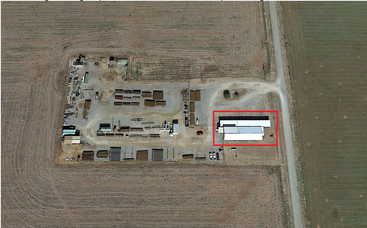
Image showing the parcel after the work had been completed (Image Date – 11/19/2014)
