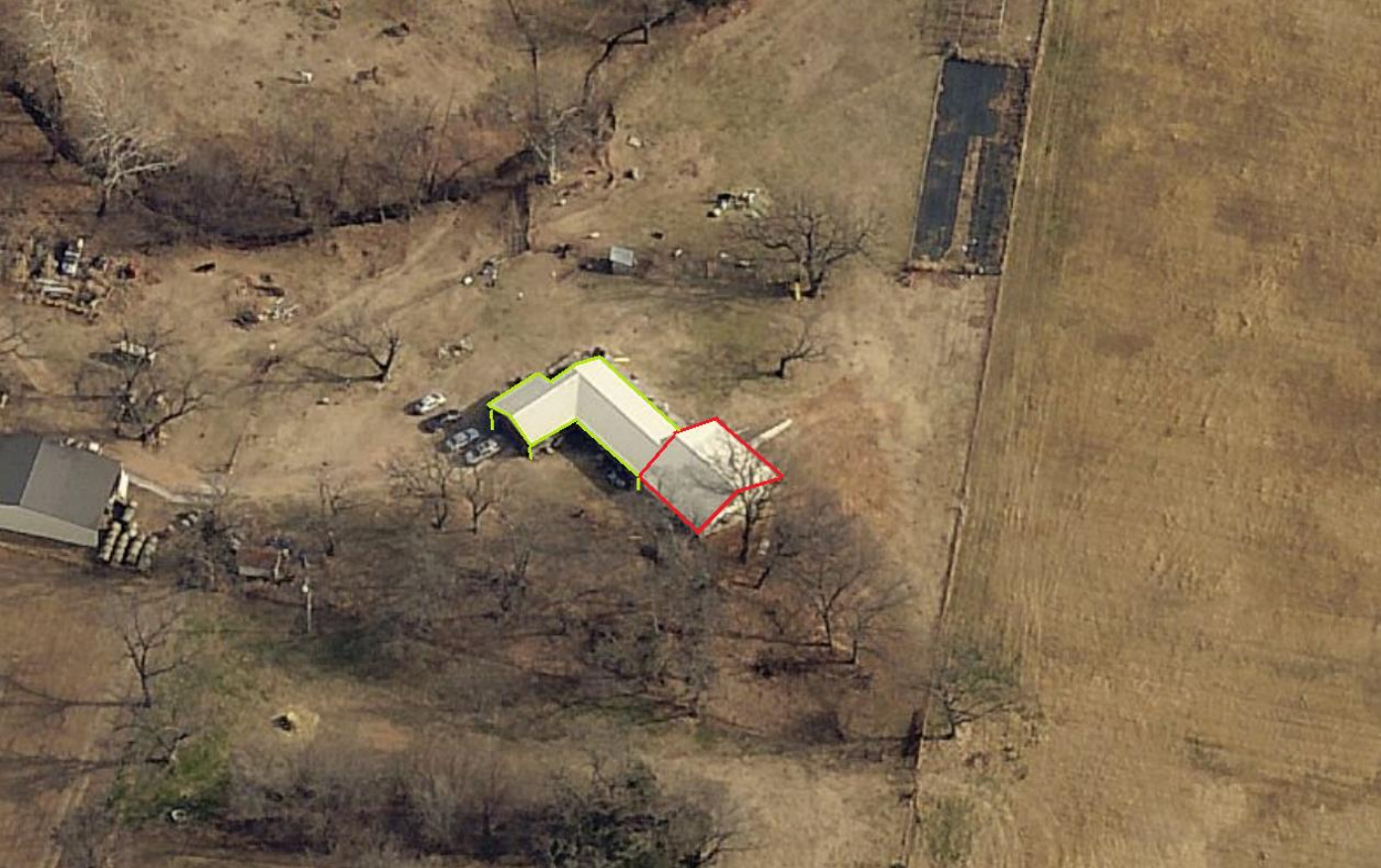
Image of the parcel following the construction of the extension (Image Date – Dec 2017)
