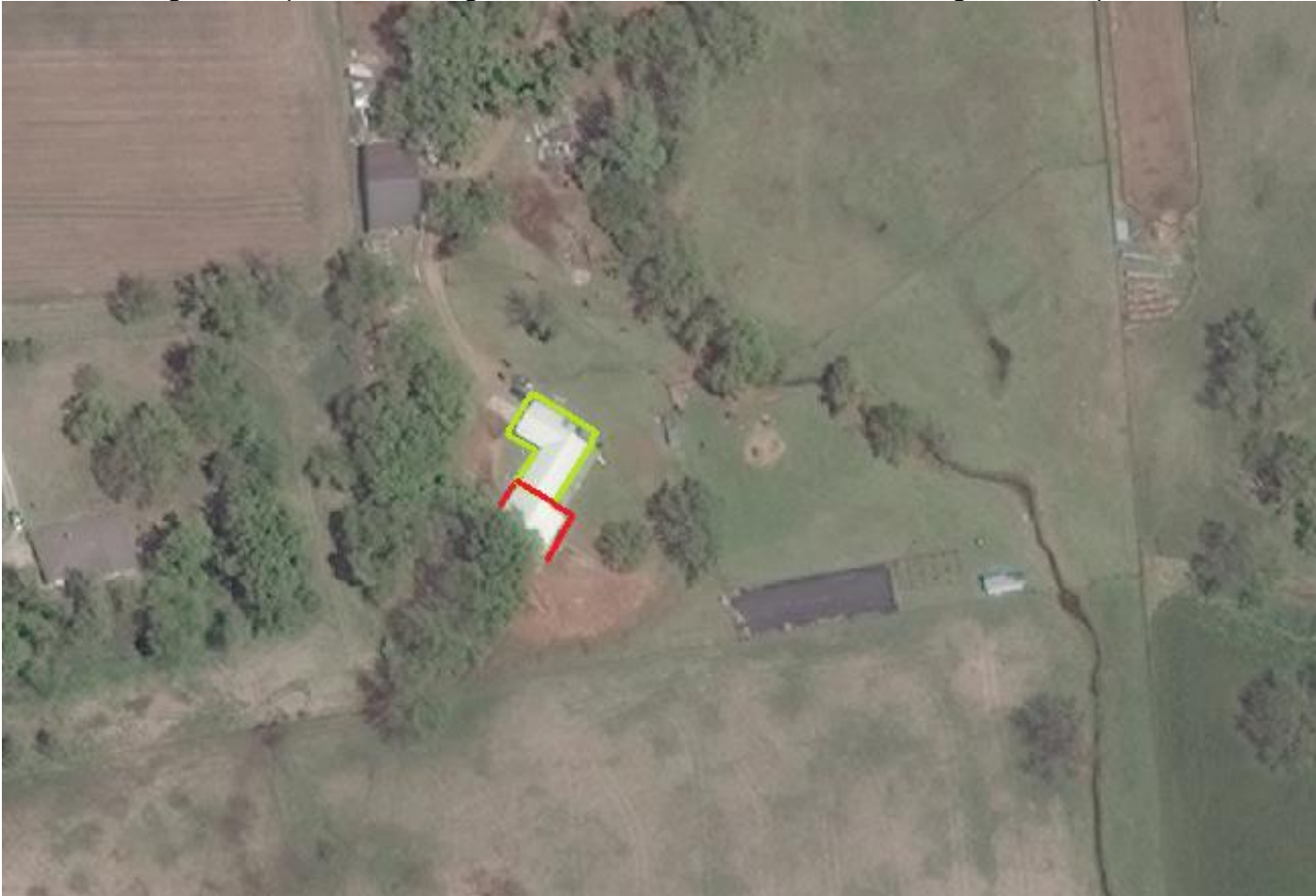
Image of the parcel following the construction of the extension (Image Date – April 2016)
